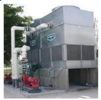
result of several water based cooling systems being decommissioned due, in part, to the high cost of maintenance and water treatment involved and also as a result of the continuing development of quieter, more energy efficient, dry ventilation systems.
